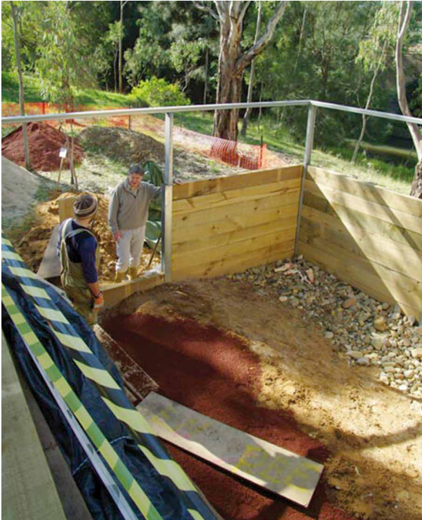
Figure 1 Laying the foundations: The Palaeolithic layer in the TARDIS.
