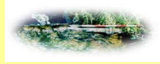
The 6 inch iron water pipe was imported from Scotland and joined in sections
