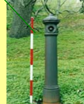
Drinking fountains such as this were located at intervals along the route of the pipeline
