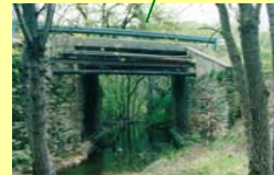
White's bridge, Brownhill Creek
